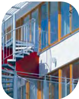
Pilkington Insulight™ Protect – Eko-Park Cameratta, Warszawa
